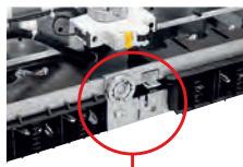
Withdrawable unit coding on the unit
